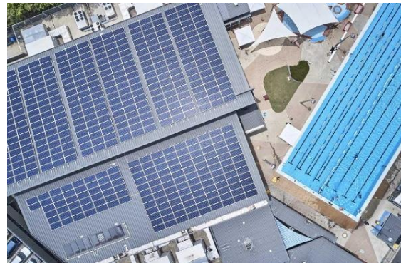
TWEED REGIONAL AQUATIC CENTRE SOLAR
